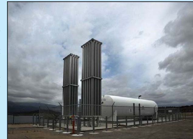
Casitas Municipal Water District installed a new hypolimnetic oxygenation system during September of 2015 to help minimize water quality problems in Lake Casitas.
